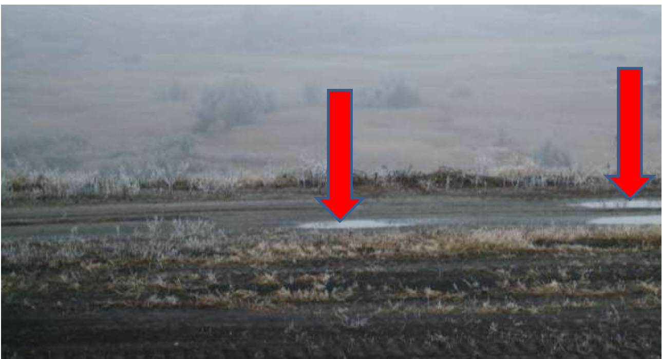
Figure A8.6: The third upper ledge of the tailings dam. Excessive waterlogging of the dam, atmospheric precipitation is not absorbed (View from the second ledge)
