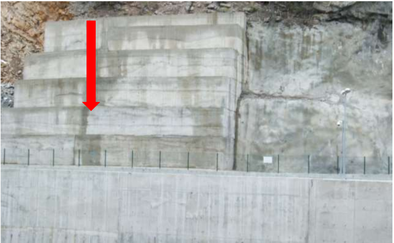
Figure A8.29: Concrete retaining wall prevents from slipping the dam
