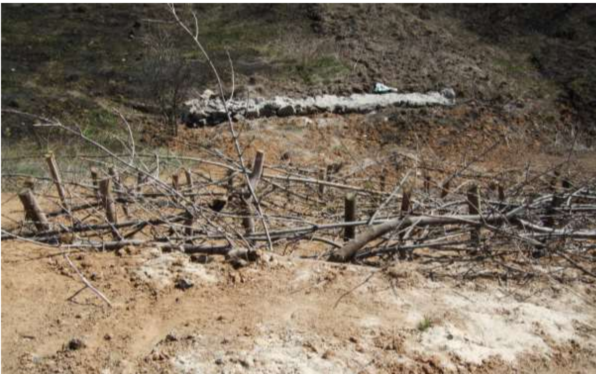
Figure A8.24: The external slope of the dam of an abandoned TMF. The wooden pile series indicate implicitly at a landslide occurred
