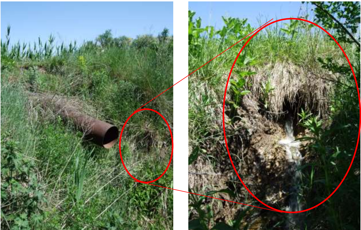
Figure A8.8: External slope of the dam. Water leaks and flows aside the spillway
