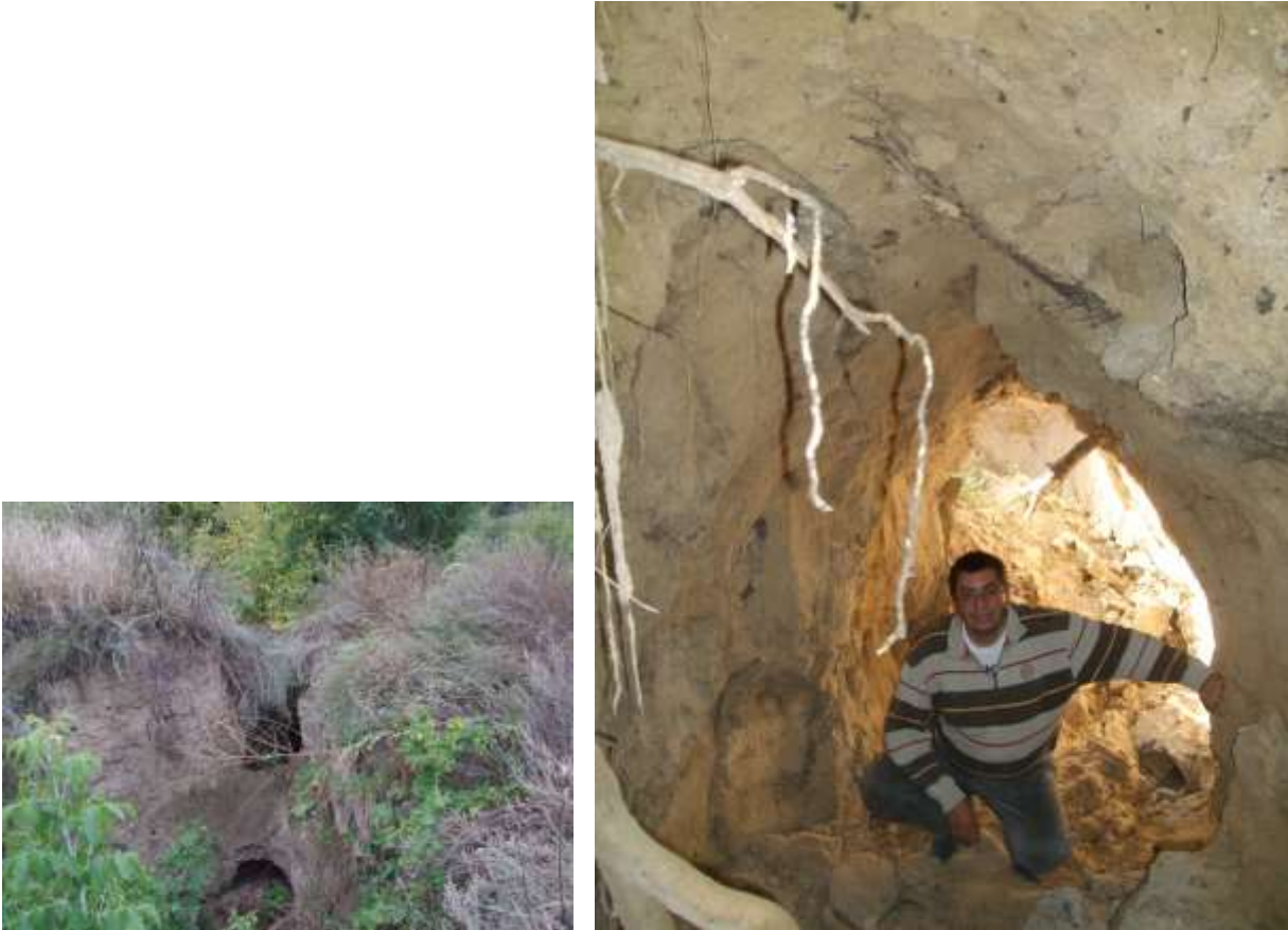
Figure A8.20: The crest of the tailings dam. Salt water accumulation in a poodle on tailings material may lead to suffusion in the dam body
