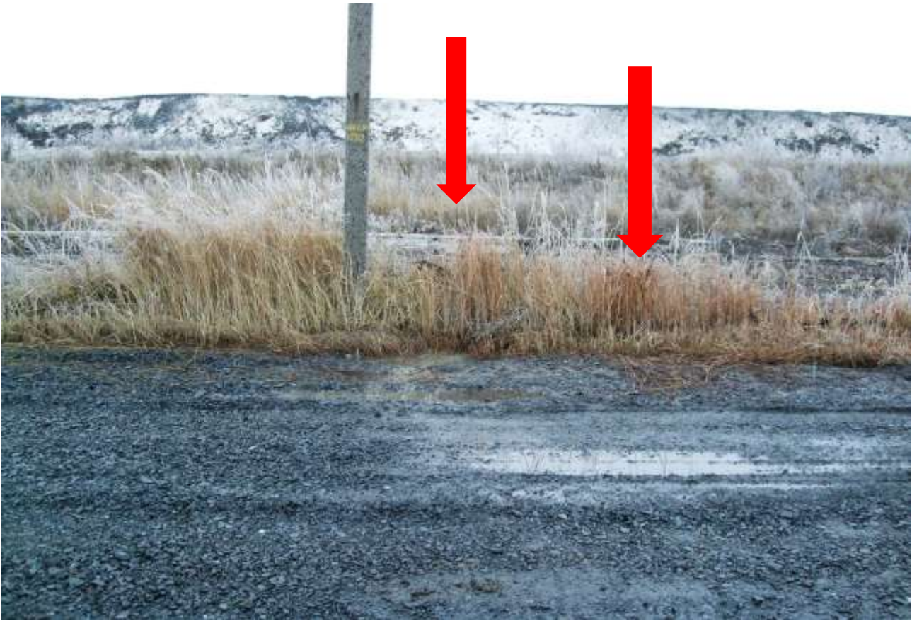
Figure A8.8: External slope of the dam. Water leaks and flows aside the spillway
