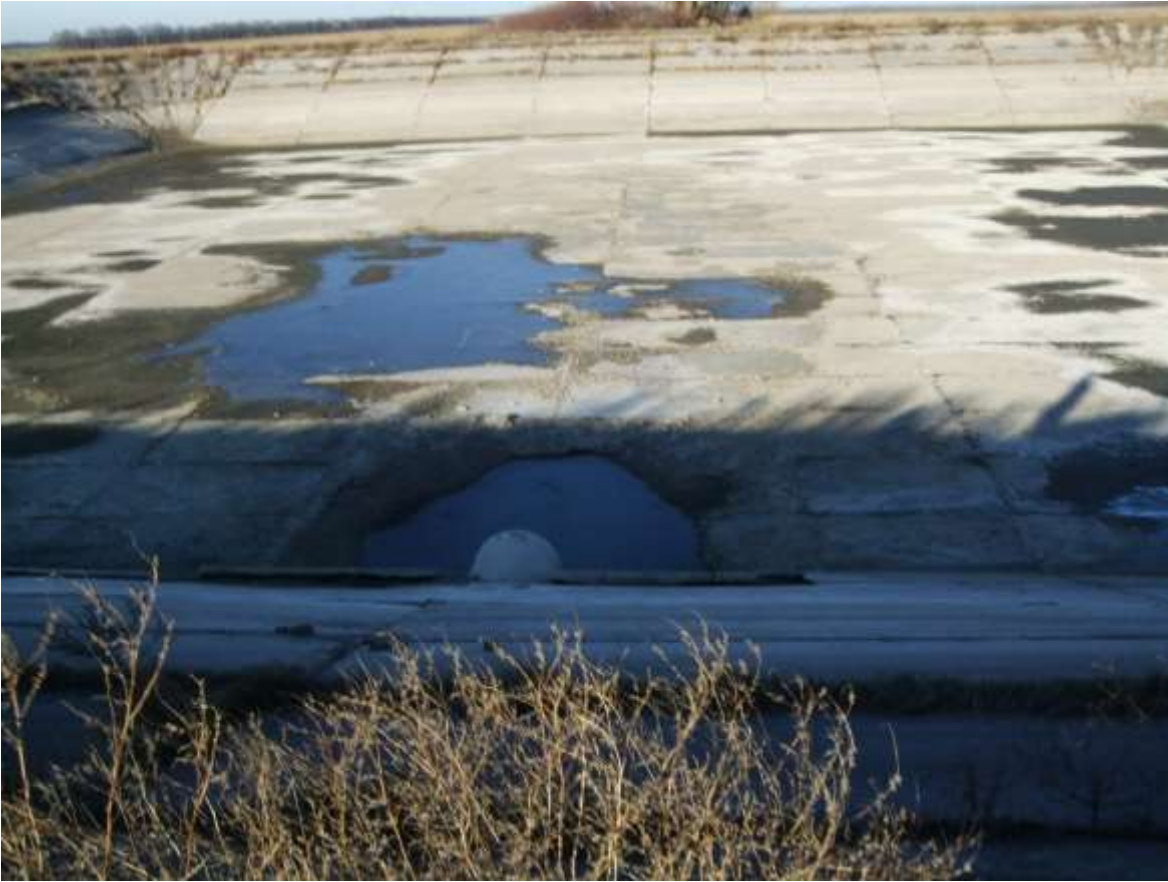
Figure A8.38: Measure 34C. Elaborate technical measures for phyto-rehabilitation of the TMF site. Biological plateau is installed for drainage water treatment (View from the tailings dam)
