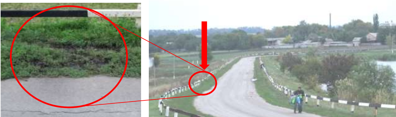
Figure A8.26: External slope of the tailings dam. A rickety road bump and a breakaway in this place implicitly evidence the emerging landslide
