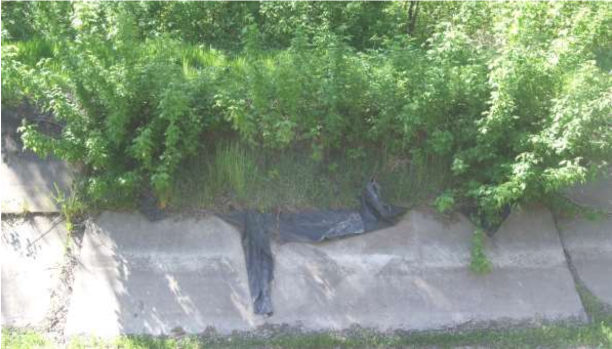
Figure A8.14: Bottom inner part of the tailings dam. Breakthrough of a waterproofing due to destruction of lining.
