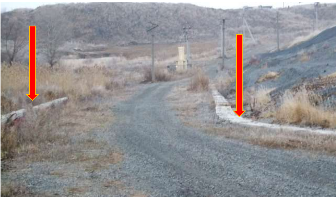
Figure A8.34: Measure 21G – Create or repair the upper ditch to reduce surface water run-off into the tailings pond. Drainage concrete gutters are installed to catch water from the dam
