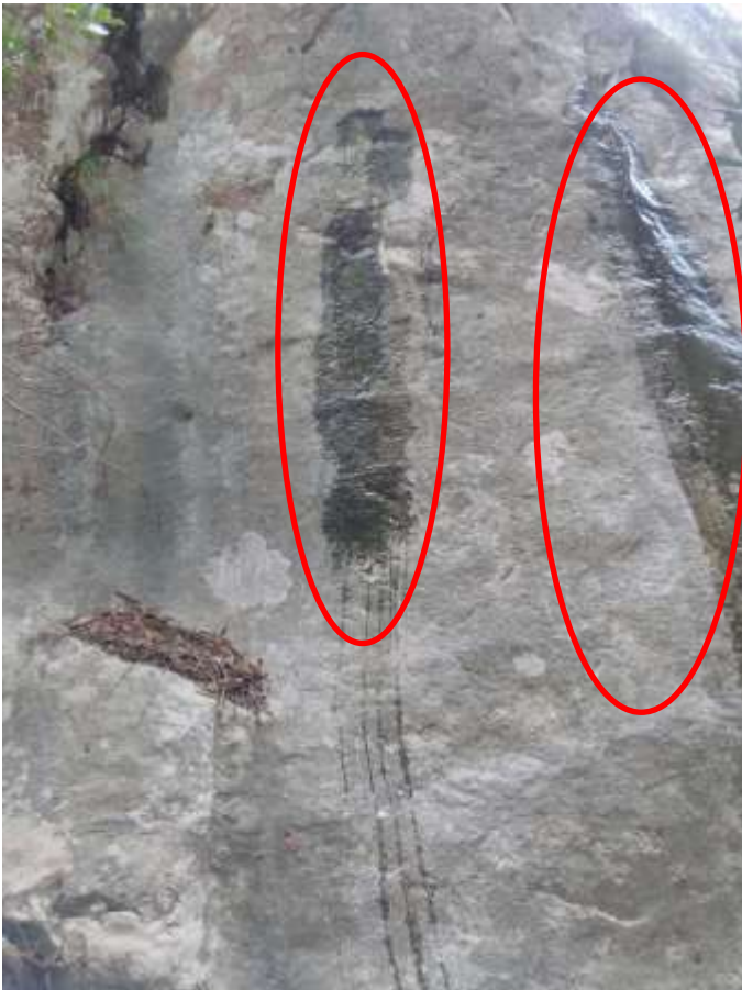
Figure A8.10: Concrete tailings dam. Seepage through the pores in the monolith is visible as "tears".
