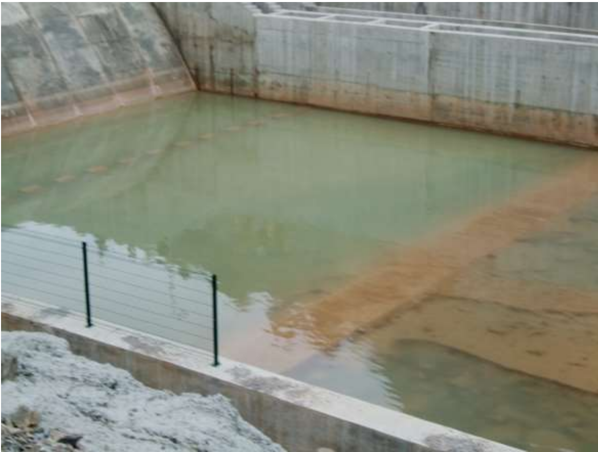
Figure A8.34: Measure 21G – Create or repair the upper ditch to reduce surface water run-off into the tailings pond. Drainage concrete gutters are installed to catch water from the dam
