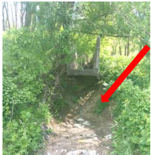
Figure A8.22: Upland drainage ditches and trays. Improper drainage of the tailings causes floor erosion of the talweg of a gully/ravine. The drainage system may be destroyed with further development of erosion
