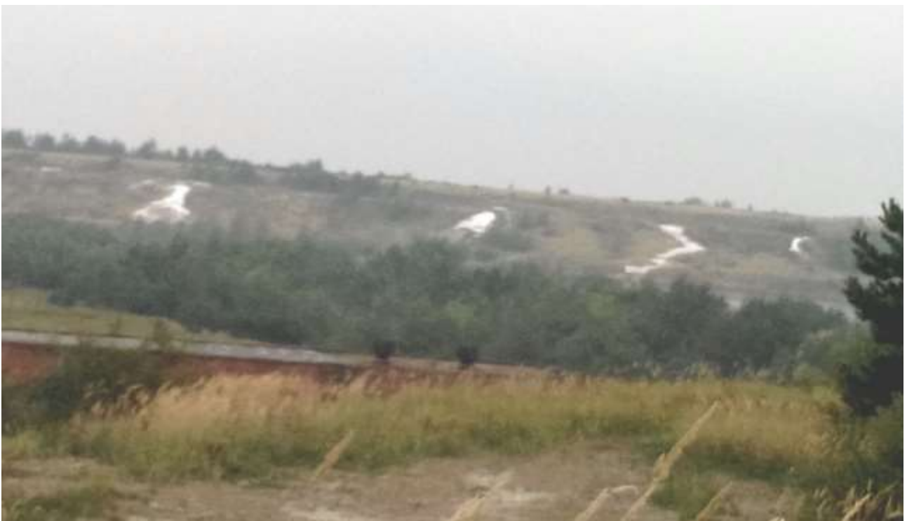
Figure A8.12: External slopes of the tailings dam. Salt is deposited on the slopes as a result of seepage of mineralized tailings water through the dam body (Photo taken at the TMF near Kalush, Ukraine)
