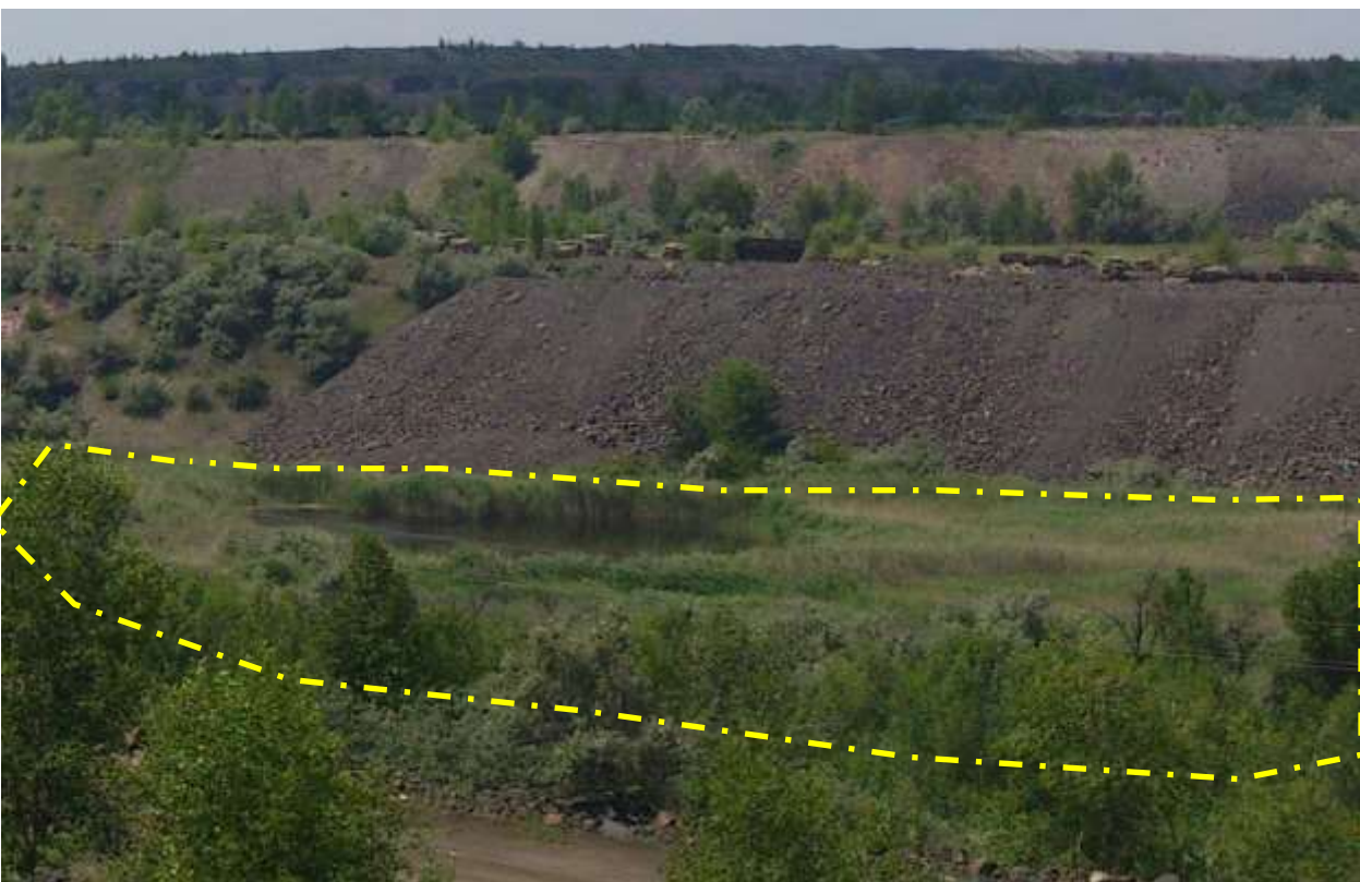
Figure A8.38: Measure 34C. Elaborate technical measures for phyto-rehabilitation of the TMF site. Biological plateau is installed for drainage water treatment (View from the tailings dam)
