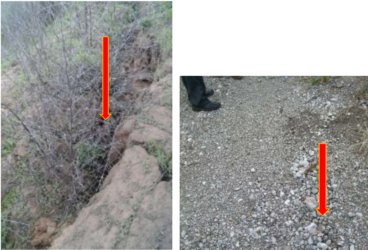
Figure A8.26: External slope of the tailings dam. A rickety road bump and a breakaway in this place implicitly evidence the emerging landslide
