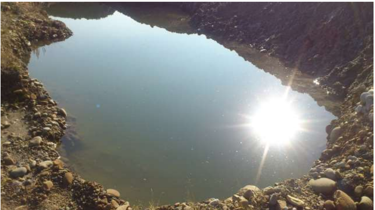
Figure A8.20: The crest of the tailings dam. Salt water accumulation in a poodle on tailings material may lead to suffusion in the dam body
