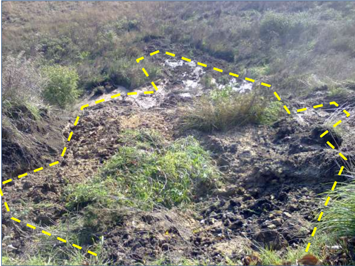
Figure A8.24: The external slope of the dam of an abandoned TMF. The wooden pile series indicate implicitly at a landslide occurred
