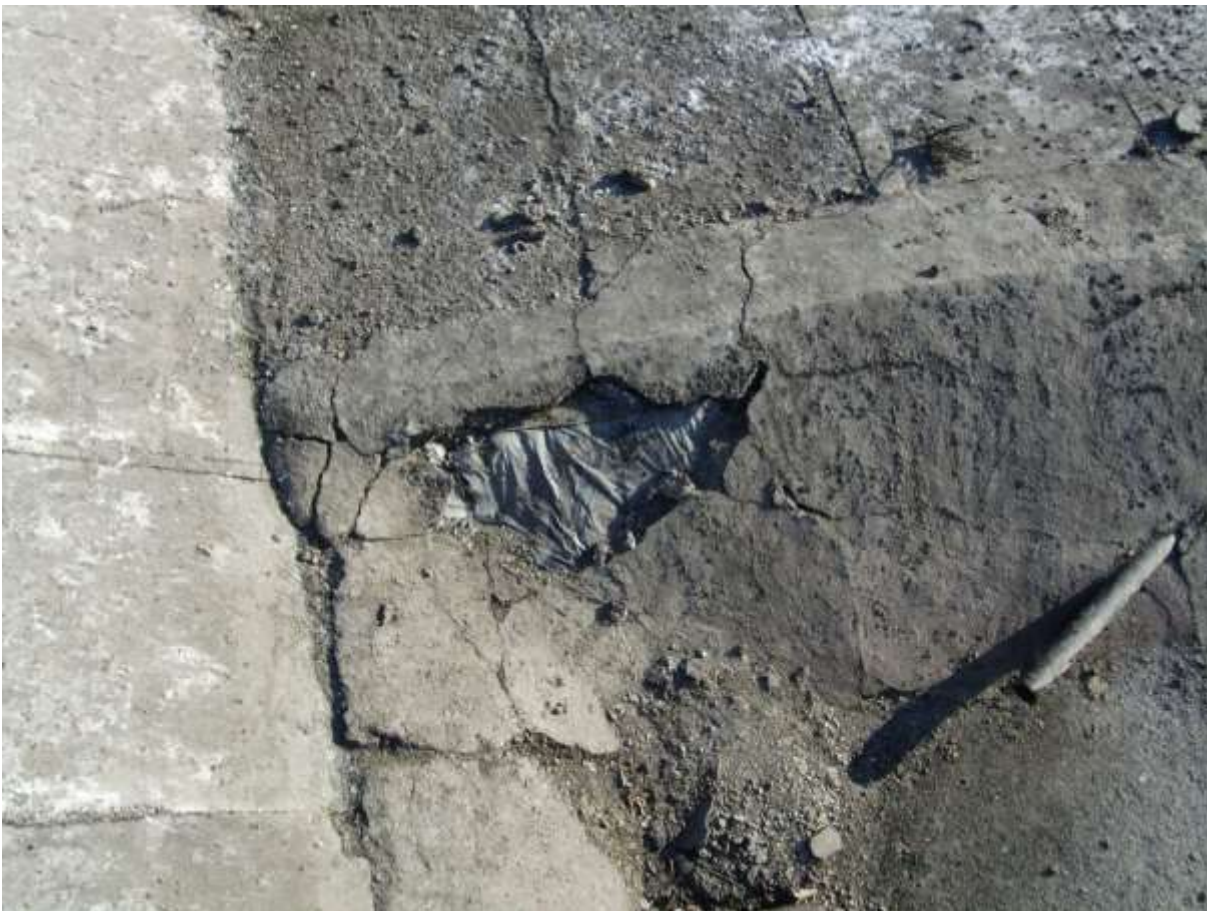
Figure A8.14: Bottom inner part of the tailings dam. Breakthrough of a waterproofing due to destruction of lining.
