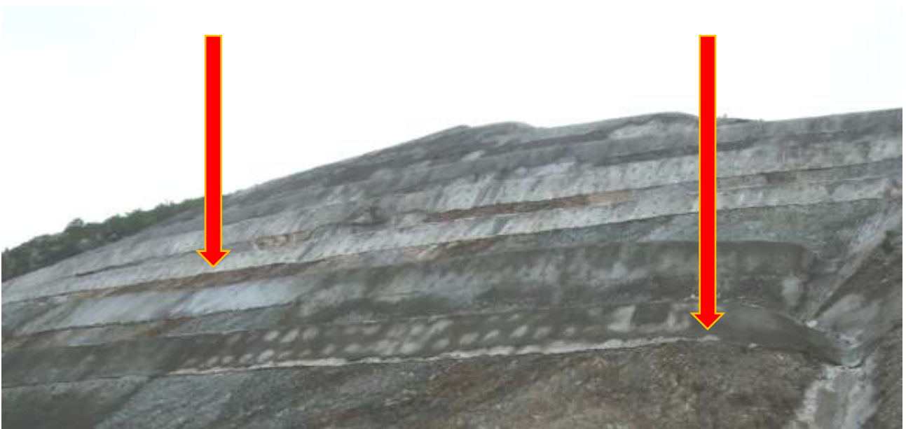
Figure A8.28: Measure 19C – Strengthen the dam using grouting and/or drainage curtains. The slope of the tailings dam has been cemented.
